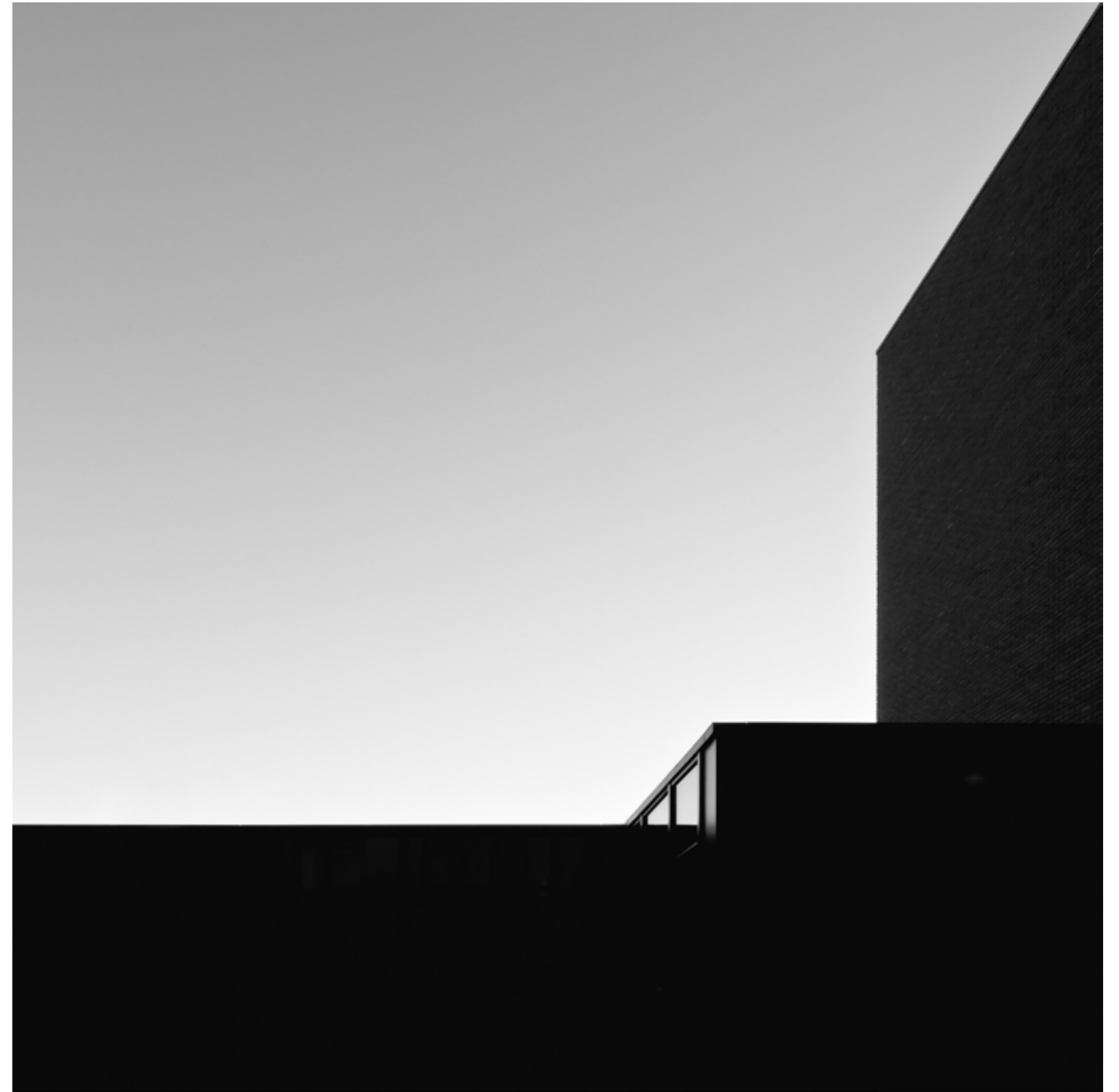
Care Center Koen Van Damme, Belgium
