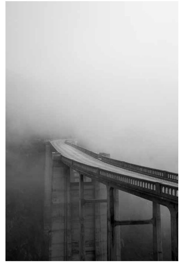
Bridge Aaron Citti, Australia
